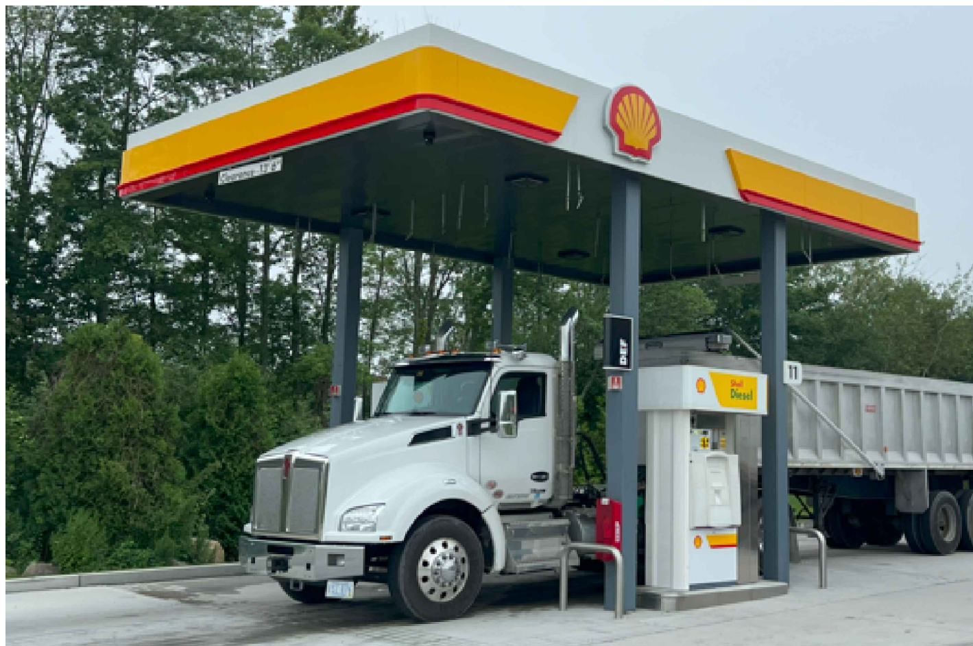
Existing Diesel Canopy
